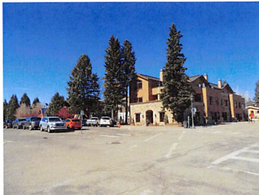
SW CORNER, EAST AVE. & 4TH ST.
