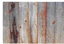
EXTERIOR FINISH 5 (EF-5): WEATHERED WOOD BOARD, VERTICAL, EXACT PRODUCT TBD
