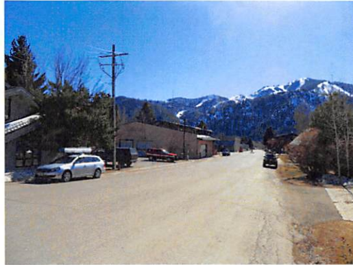
NE CORNER, FIFTH ST.
