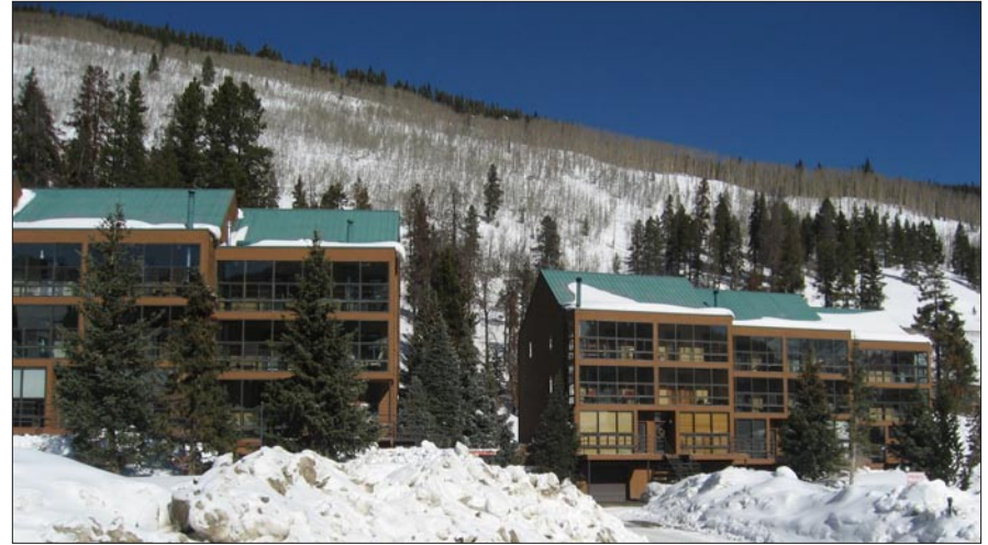
When on a sloped site, a building should reflect the change in the elevation of the site through stepped and articulated sections of the building massing.
