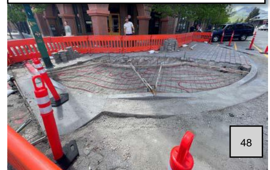
Example bulbout/ snowmelt construction
